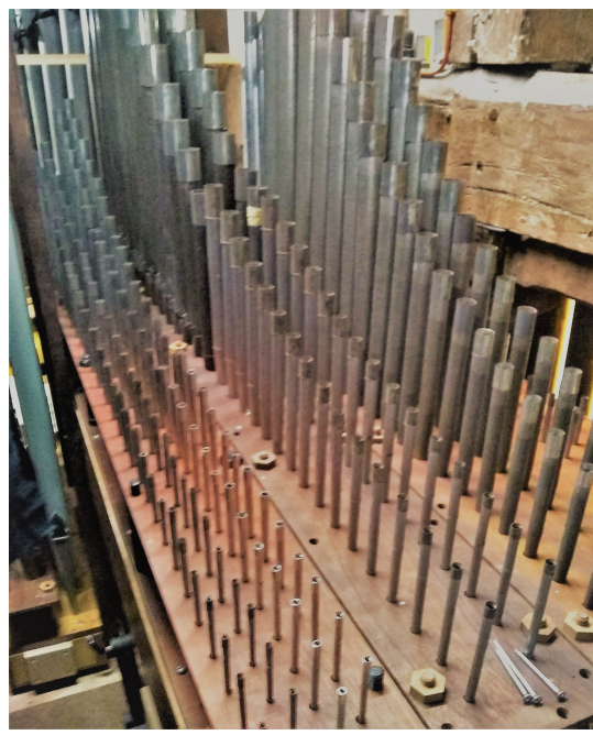
Great pipework cleaned, speech reset and re-located
