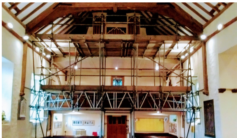
Scaffold at West end
